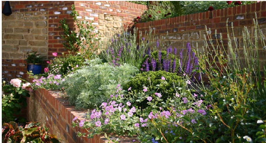
Recycled bricks - planters and retaining wall adjacent to service road
