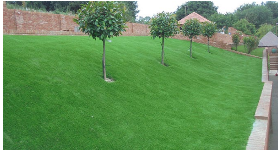
Recycled bricks - raised kerbs and retaining wall
