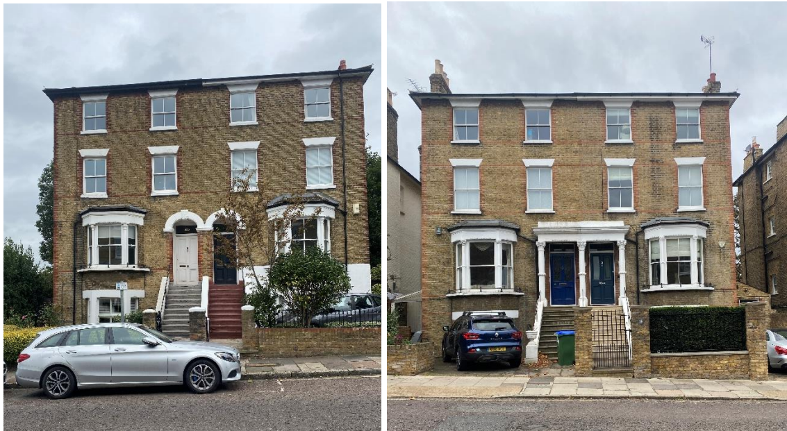
Figure 9 (left) typical pair from the eastern side of the road with arched door openings; Figure 10 (right): typical pair from the western side of Church Road with shallow flat roofed porches.
