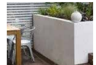
Retaining wall for level change
