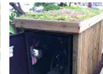
Cycle store with green roof
