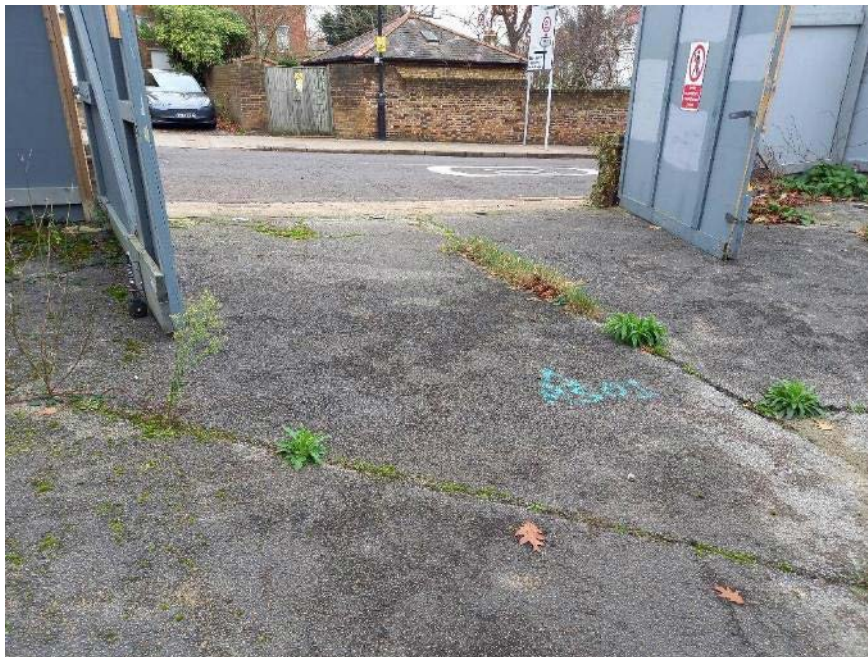
Figure 4. Area of hardstanding at the entrance to the site
