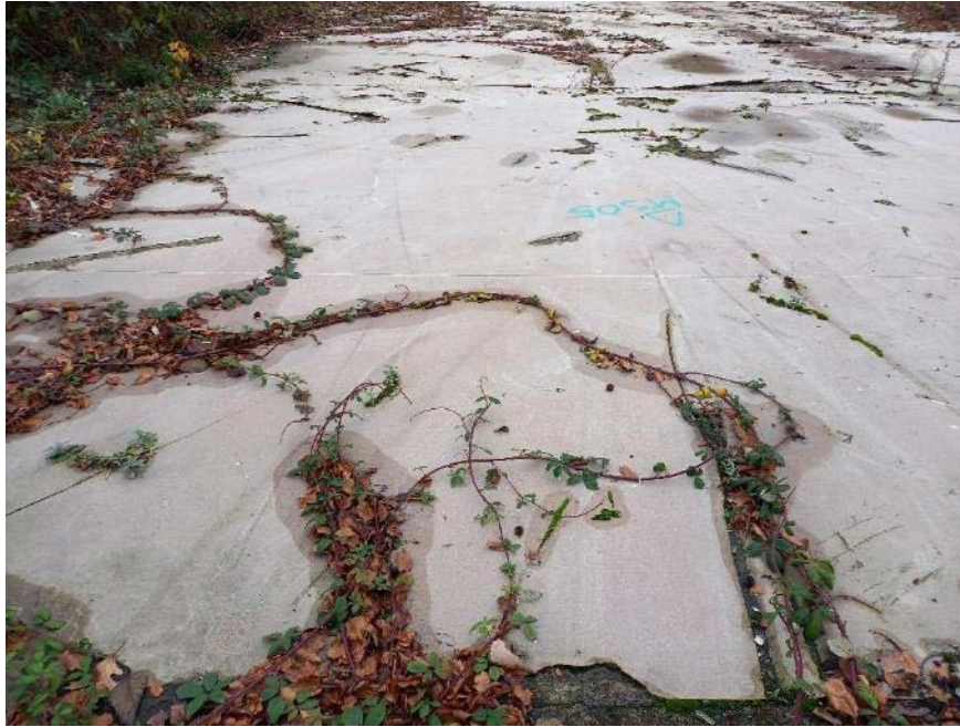
Figure 5. Area of hardstanding at the eastern side of the site
