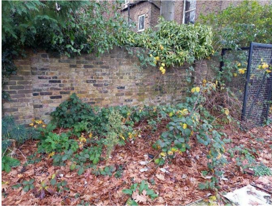
Figure 8. Area of scattered scrub along the southern boundary
