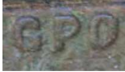
Cast iron GPO marking
