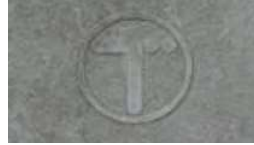
Fibreglass Telecom marking
