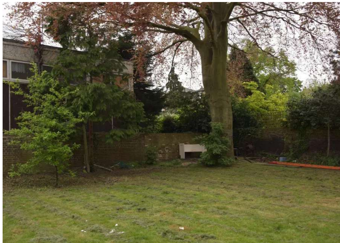
Meadows hall prior to demolition from neighbours garden
