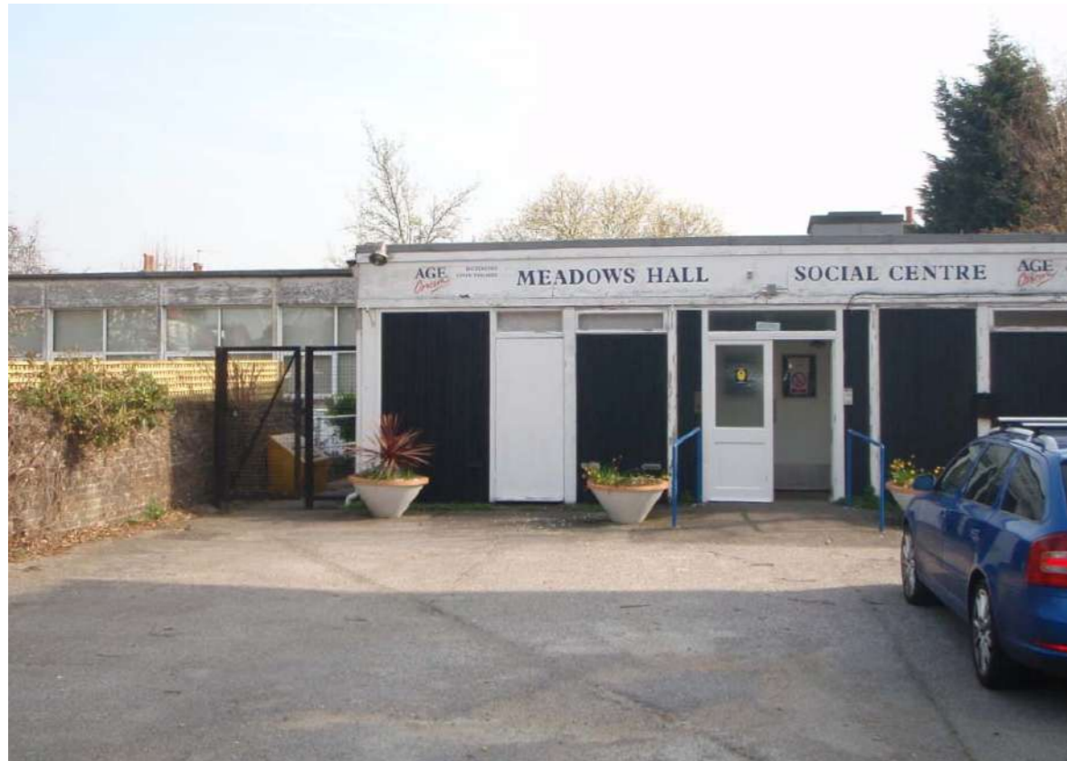
Meadows hall prior to demolition
