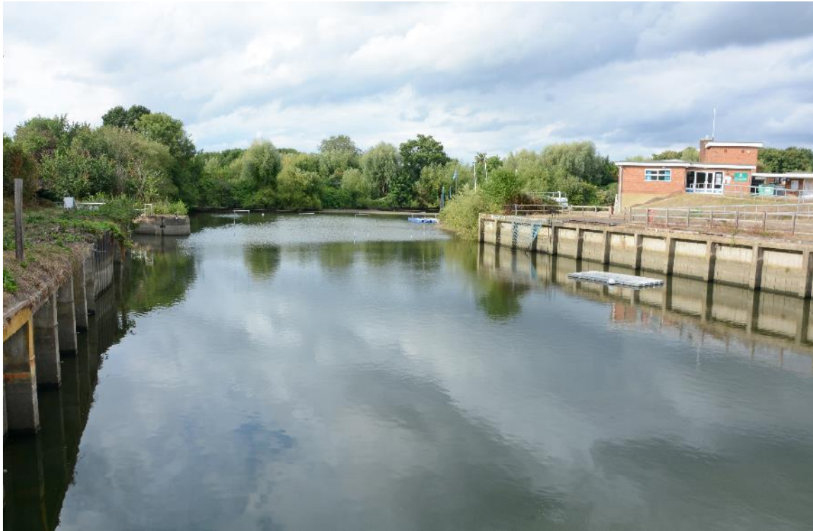
Figure 30: H: View of the early-20th century dock installed by the Ham River Grit Company, with the clubhouse to the right of frame and lock to the left. Facing N.
