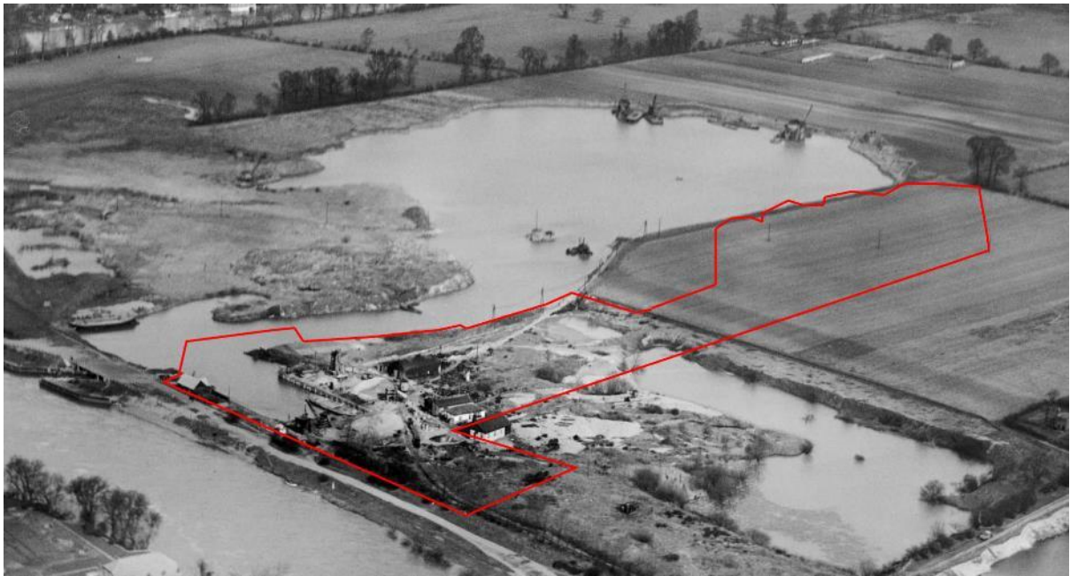
Figure 15: Aerial photograph of the study site from the SW (1927) with site approximately outlined in red. Image adapted from material held by Britain from Above (2022).
