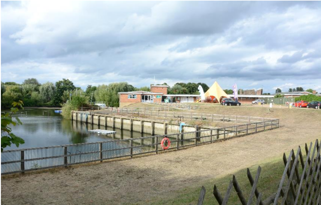
Figure 23: A: View of the dock (left) and circular driveway, looking towards the clubhouse. Facing NE.
