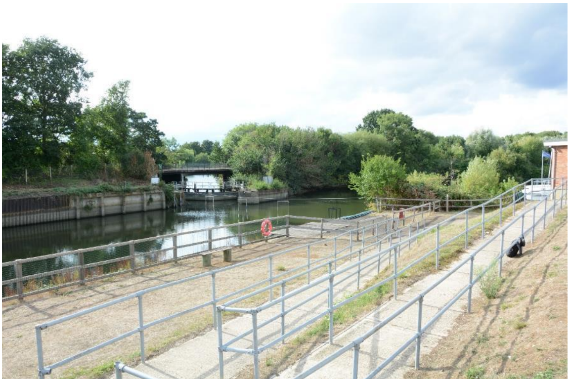
Figure 31: I: View looking across the lock towards the 1921 lock. Facing NW.
