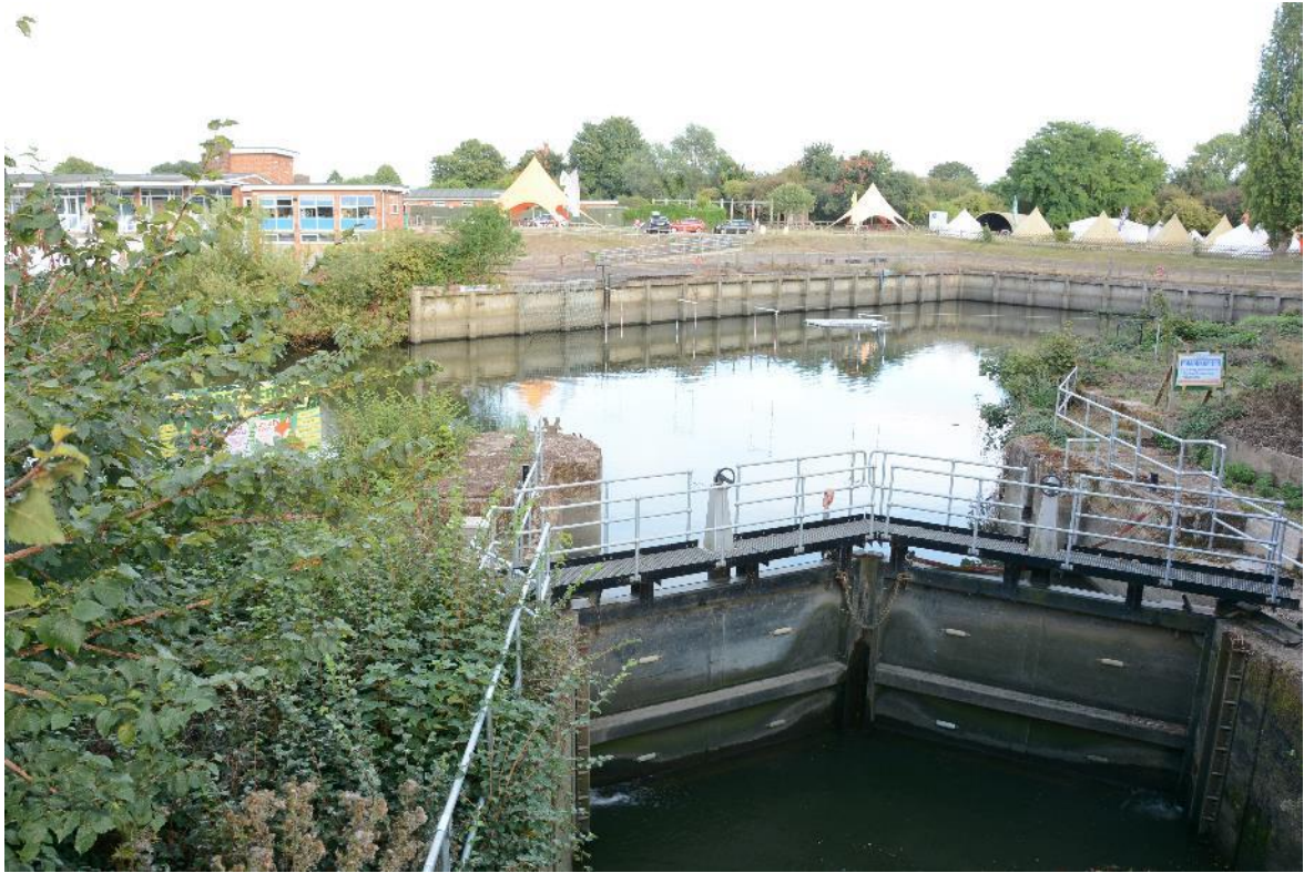
Figure 32: J: View looking from the footbridge across the lock and dock towards the main complex and camping area. Facing SE.
