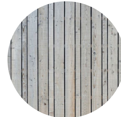
Timber Rainscreen Cladding
