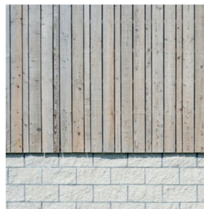
Timber Rainscreen Cladding with Stone Effect Block Upstand
