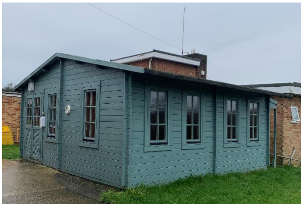
Plate 4.10: Building 2 (Wooden Cabin - North-Eastern Aspect)
