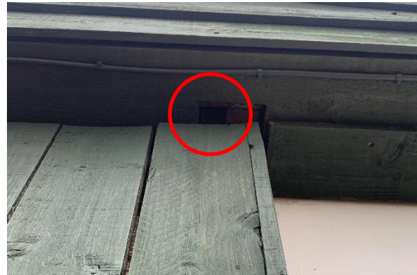
Plate 4.15: Loose Fitting Joins (Southern Aspect)
