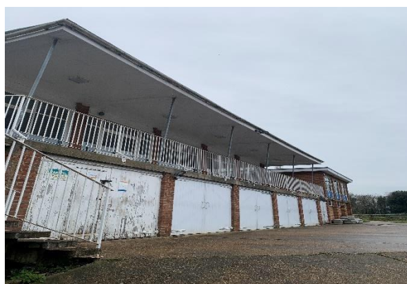
Plate 4.2: Western Elevation Of Building 1 (Main Building)
