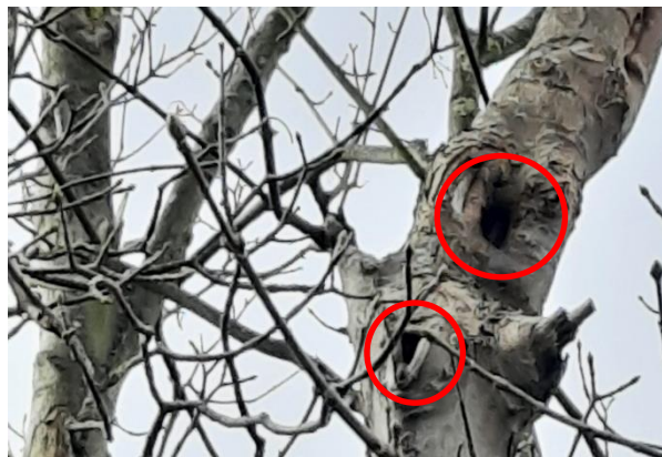
Plate 4.26: T70 Knot Holes At 5m.
