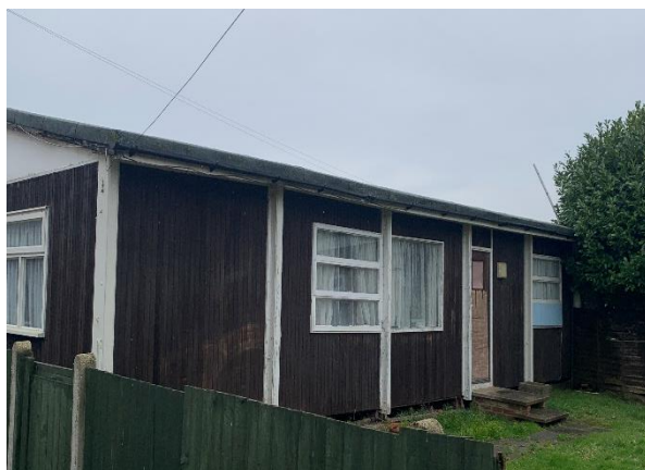
Plate 4.19: Building 4 (Cedar House)
