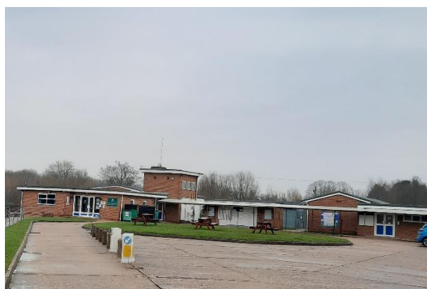
Plate 4.1: Building 1 (Main Building – Southern Elevation)
