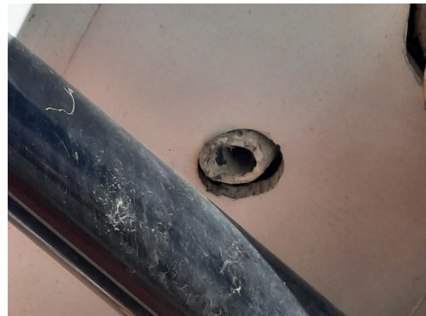
Plate 4.23: Pipe Hole (Southern Aspect)
