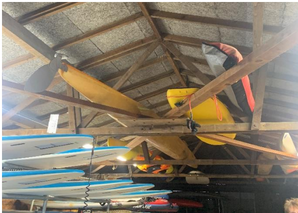
Plate 4.17: Interior of Building 3
