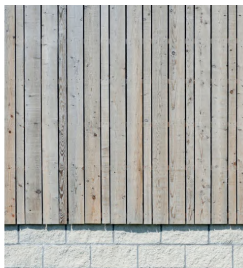
Timber rainscreen cladding with stone effect block upstand
