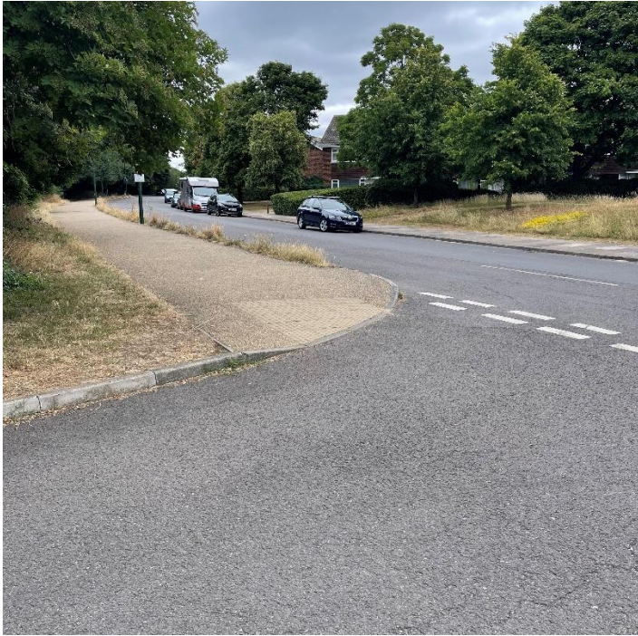
Photo 5.5 Tactile paving and dropped kerbs to cross TYM access
