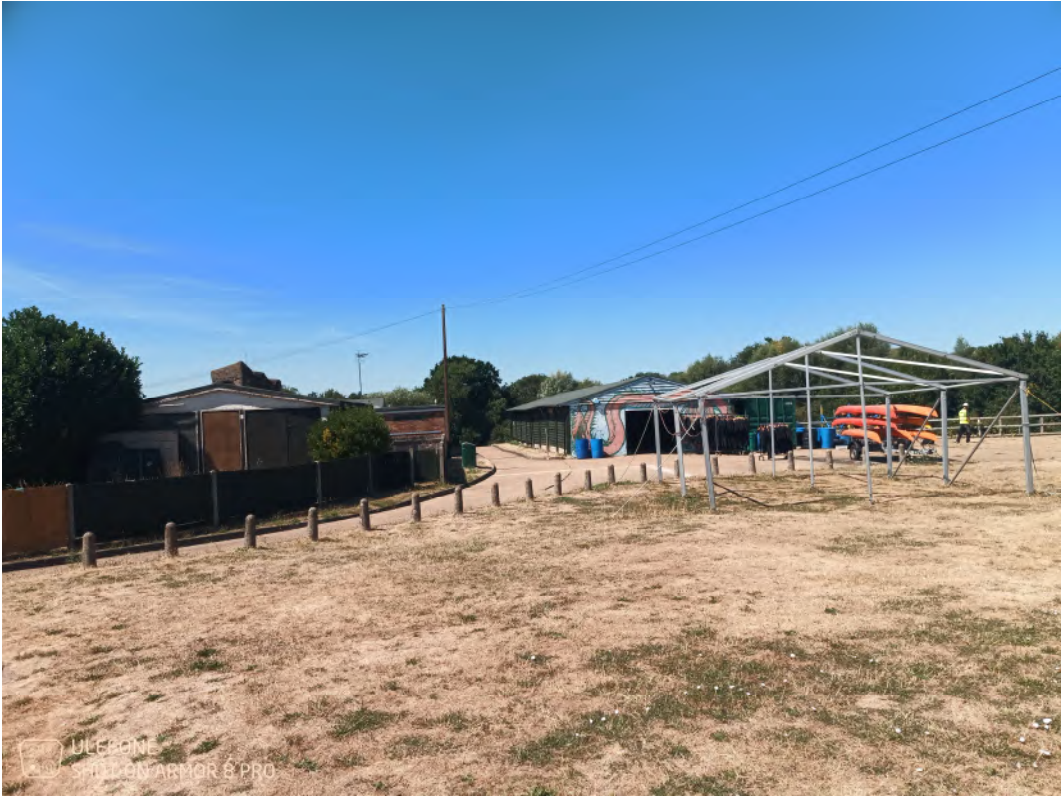
Photo 3: Looking northwest along the northern side of TYM complex.
