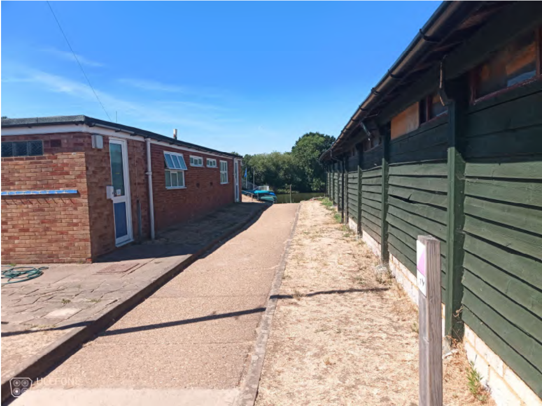
Photo 10: General photo of buildings within TYM complex.
