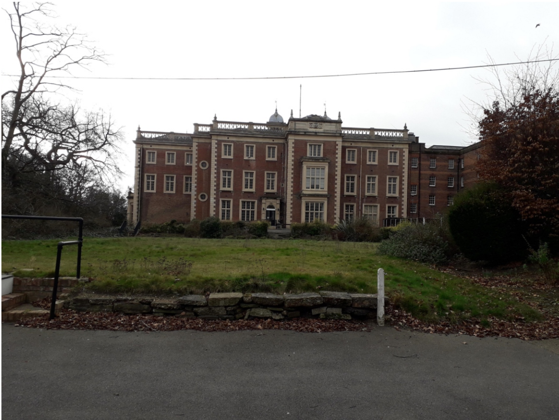
Fig 18 Kneller Hall main building, looking south (MOLA photo, 03-02-2022)
