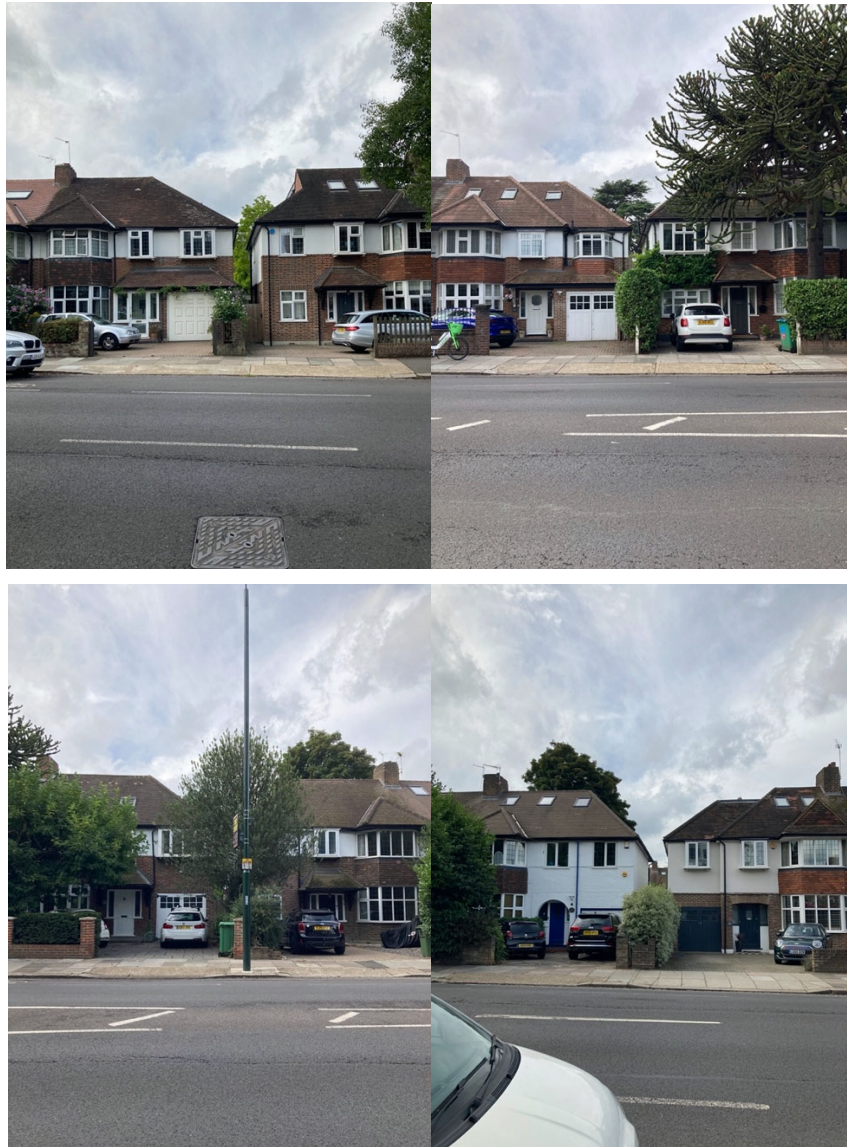
Figure 2. Neighbouring properties' side extensions. (From upper left: #65, #69, #73, #77 Twickenham road)
