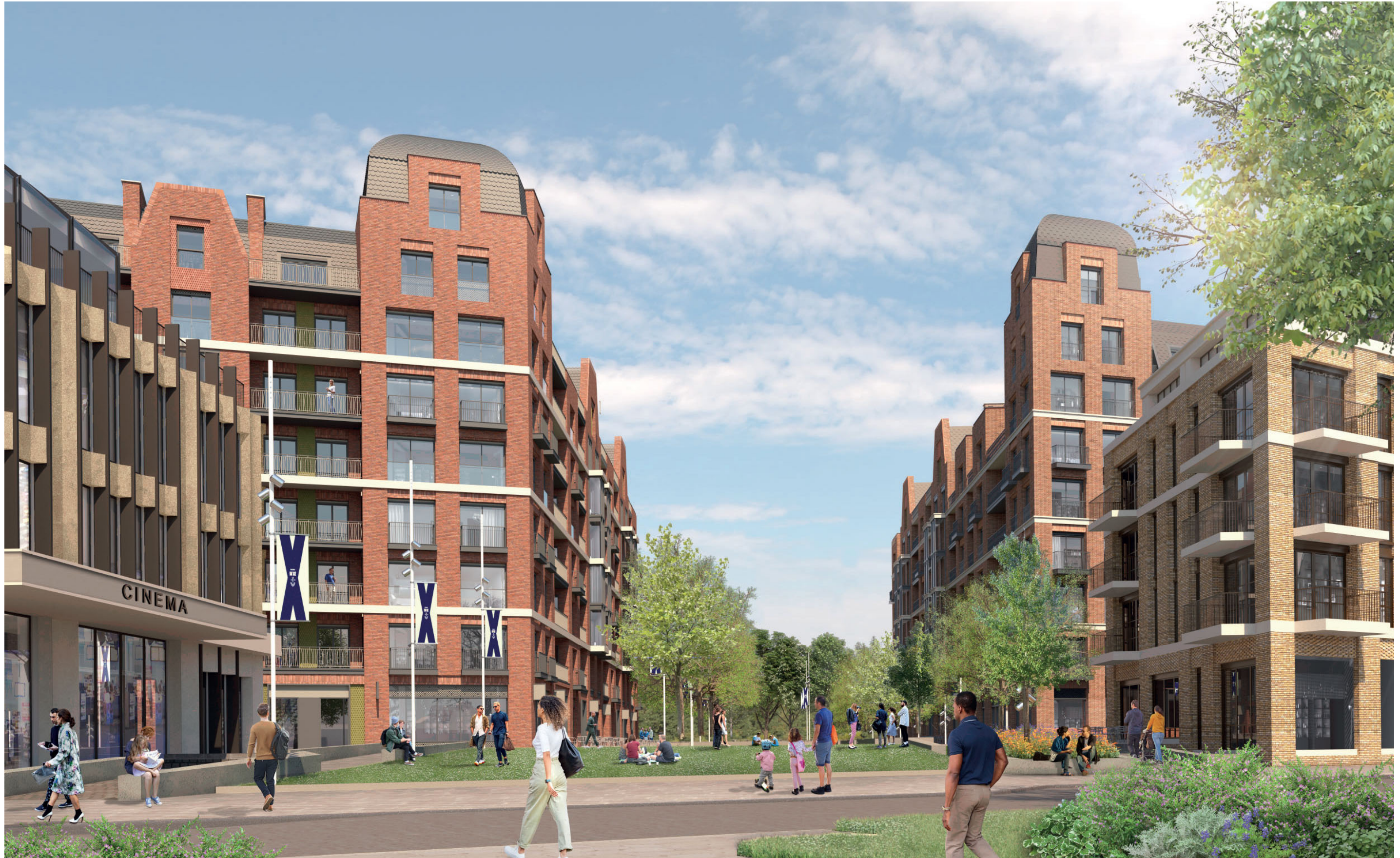
March 2022 Proposed Scheme: View from crossing on Lower Richmond Road looking towards the Green Link
