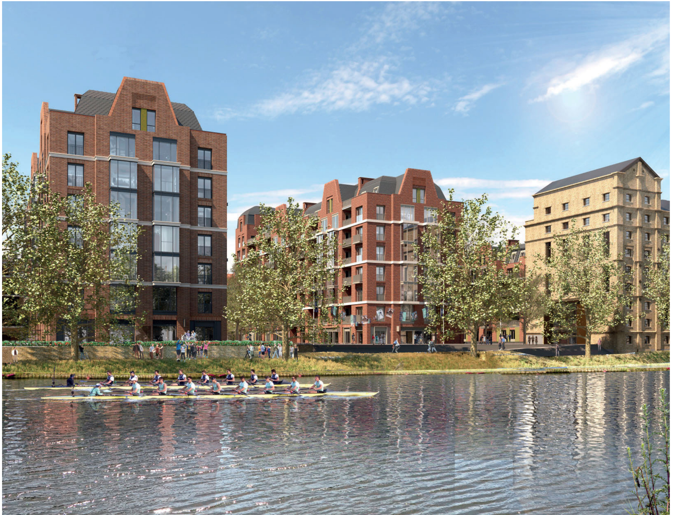
March 2022 Proposed Scheme: View from River Thames looking towards new riverside square
