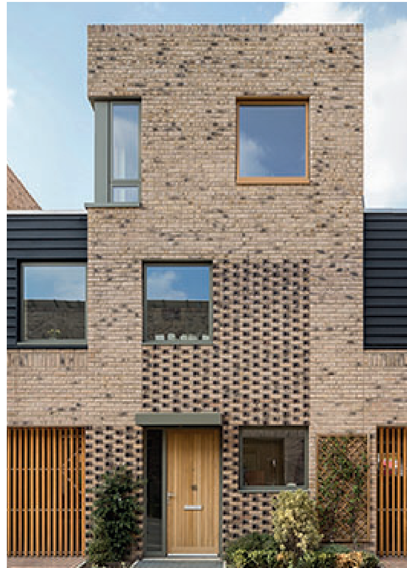
Example of timbers secondary elements only
