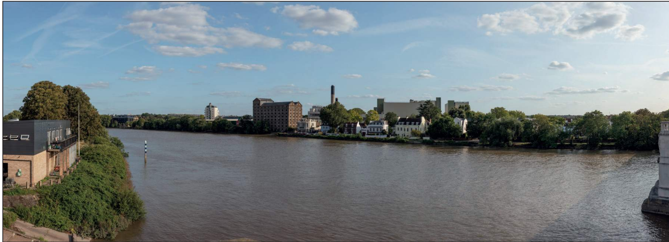
Viewpoint 4: Existing view from the northern end of Chiswick Bridge, looking south across the River Thames towards the Site.
