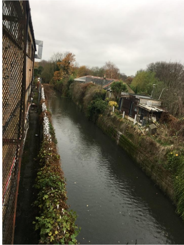
Photo 1: View of Exiting Riverside Habitat showing channelised with concrete sides with limited terrestrial ruderal vegetation
