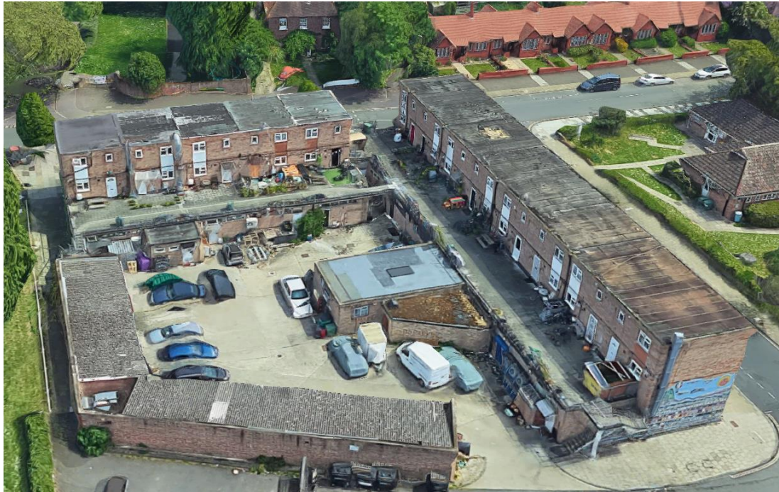
Figure 2 - Image of 65-77 Ham Street and 2-14 Ashburnham Road's Roof Top Entrance Ways
