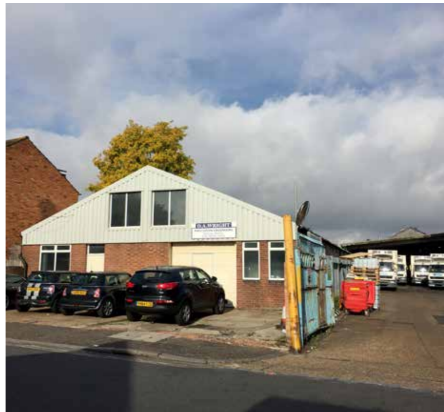
7. View looking north west of the commercial unit within site adjacent to Edwin Road entrance
