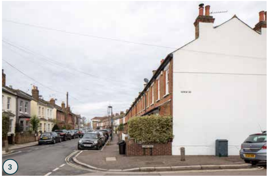
3 Western pavement of the junction between Crane Road and Edwin Road, looking north
