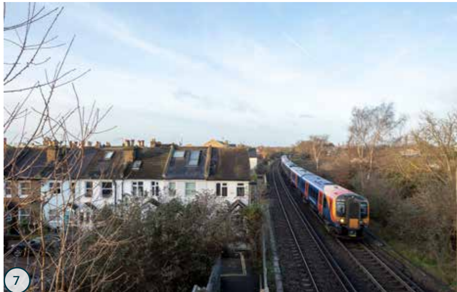
7 Footbridge crossing the railway, looking southwest
