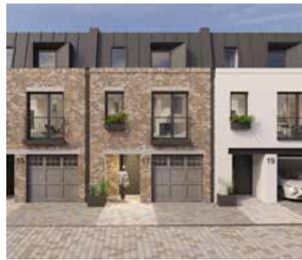
View of west terraced houses
