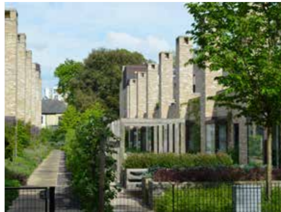
Example of pedestrian surface treatment
