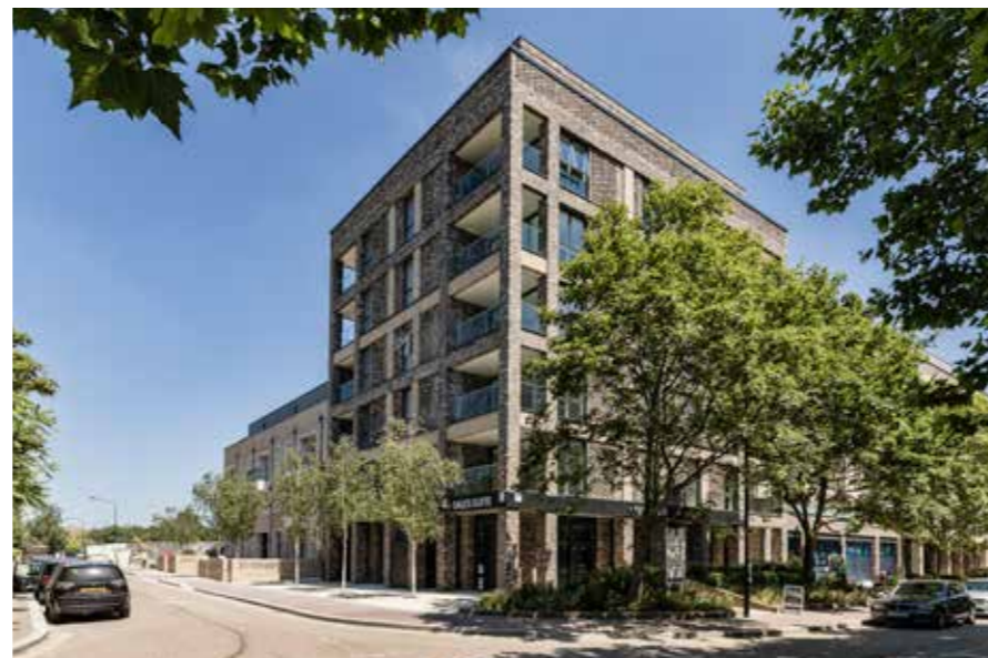
Quebec Way, Canada Water - with London Square
