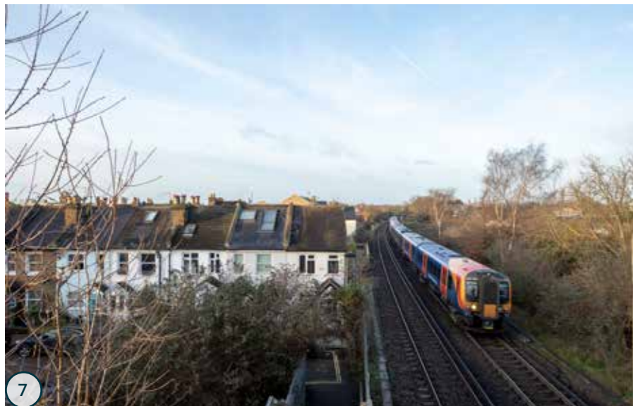
7 Footbridge crossing the railway, looking southwest
