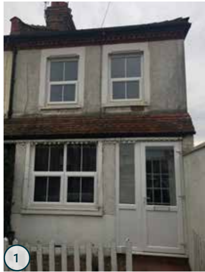
Existing house - No. 1 Gould Road
