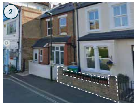
Metal fence on brick piers
