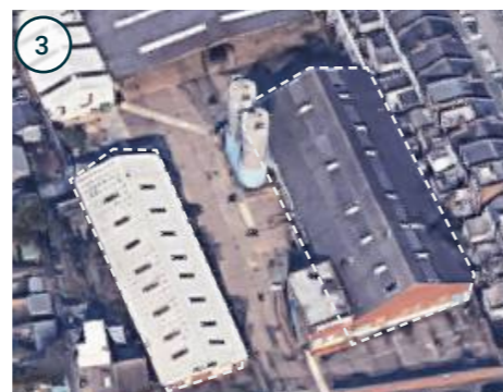
Existing site materials include white and grey metals and pitched roofs
