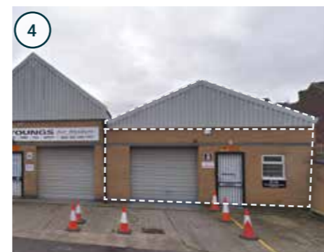
Opposite site, shows metal roof on brick walls
