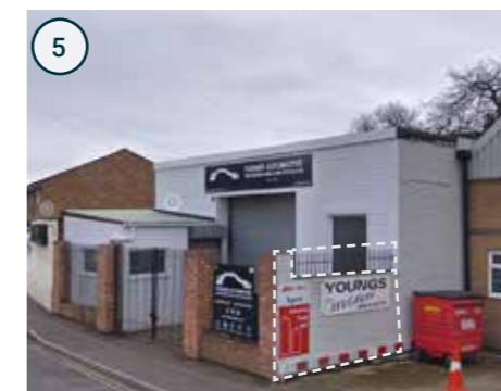
Opposite site, shows painted white bricks with metal fencing above
