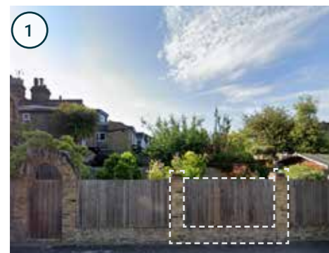
Wooden fence on brick piers
