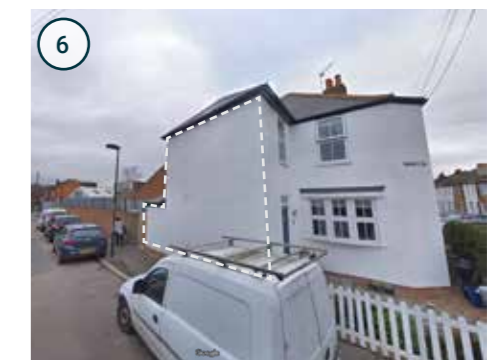
White plastered house adjacent to site
