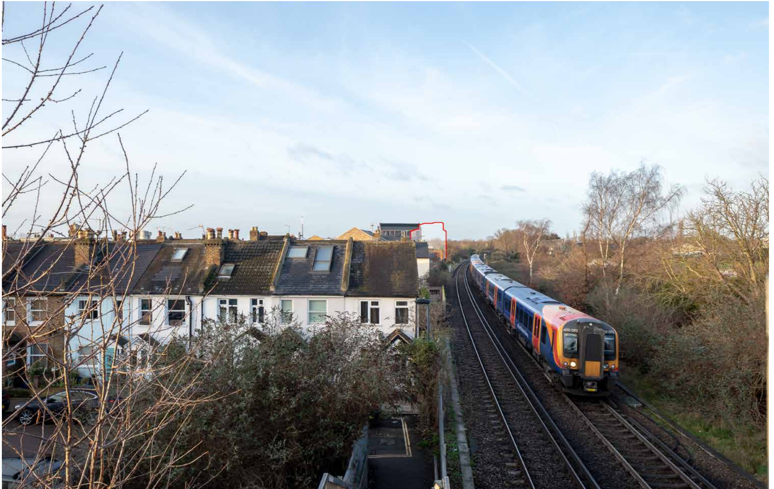
7. Footbridge crossing the railway, looking south west
