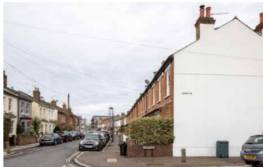
3. Western pavement of the junction between Crane Road and Edwin Road, looking north
