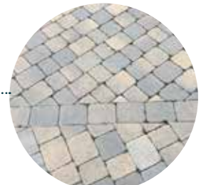
Paving setts and different tones / bands to delineate parking bays
