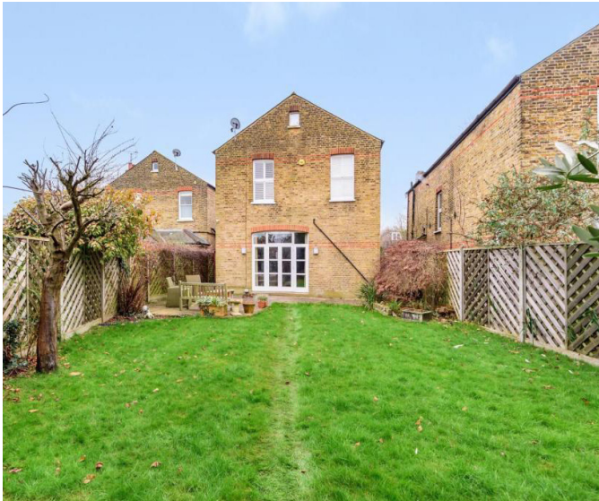
Rear elevation of 5 Cromwell Road, showing staggered relationship to neighbours
