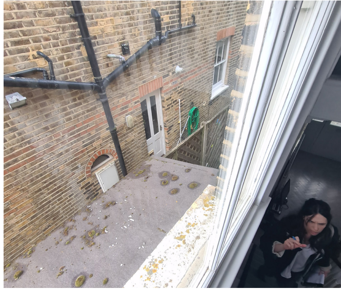
View of neighbouring no. 7 Cromwell Road and boundary
