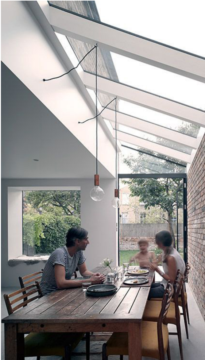
Glazed Roof to extension
