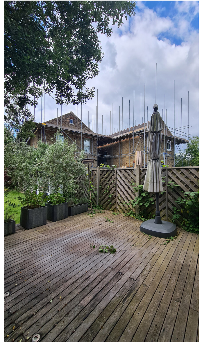
View of no1&3 Cromwell Road showing staggered building line
