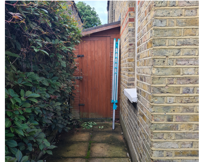
Eastern side alley way blocked by impractical long, skinny storage shed
