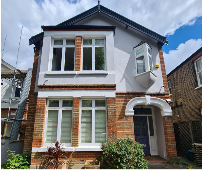
Front elevation of 5 Cromwell Road
