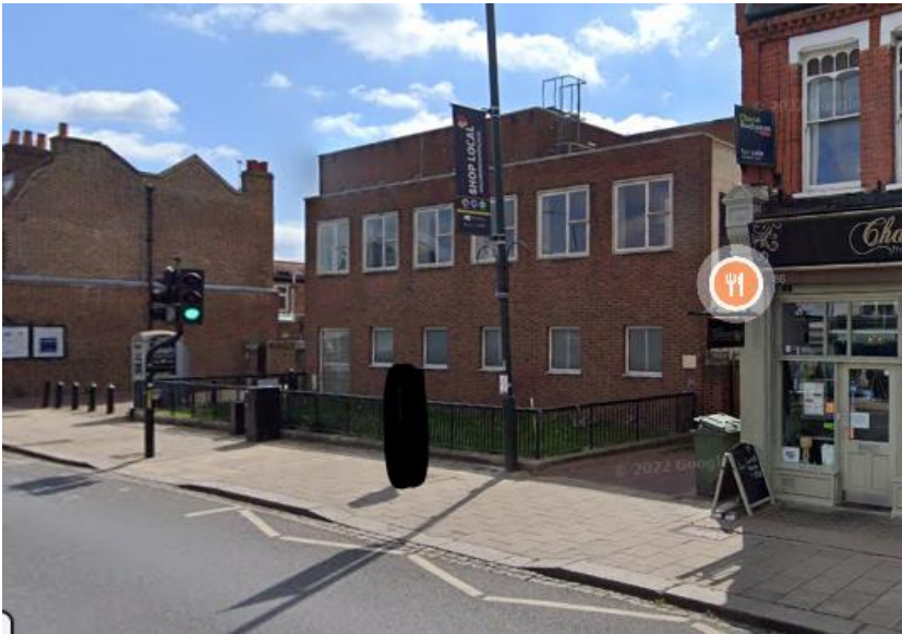
Figure 2. Telephone Exchange, High Street Teddington
