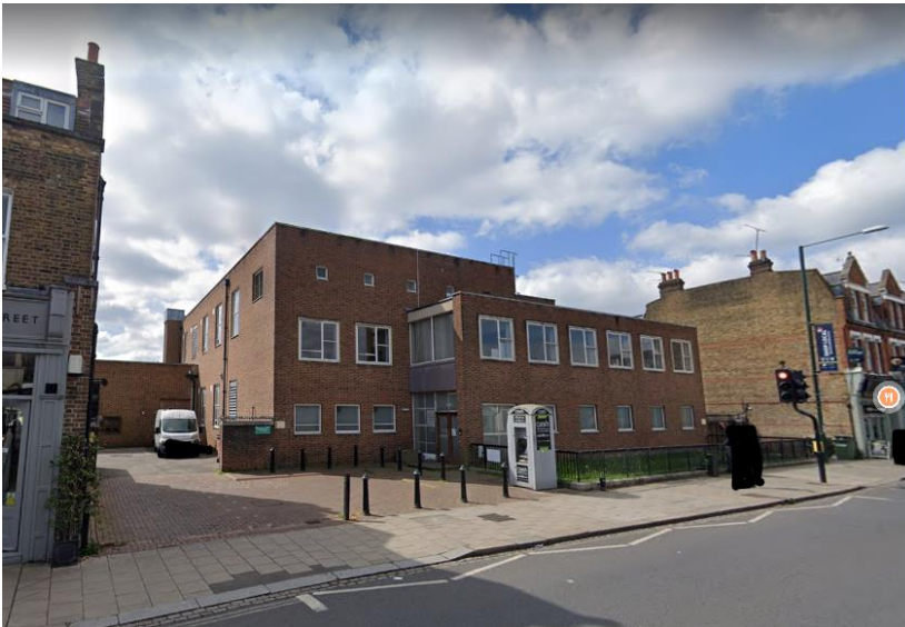
Figure 1. Telephone Exchange, High Street Teddington
