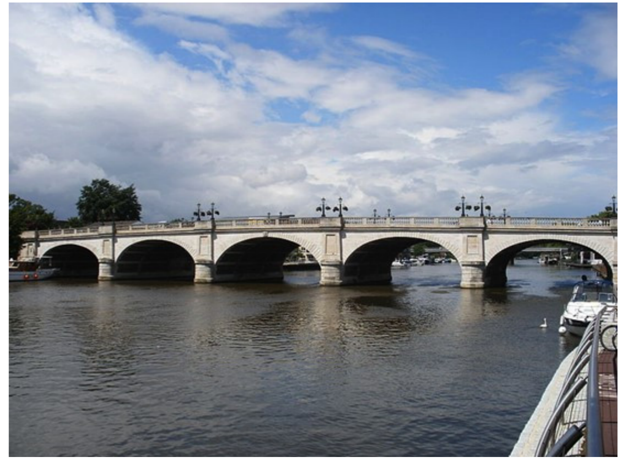
Grade II* Kingston Bridge
