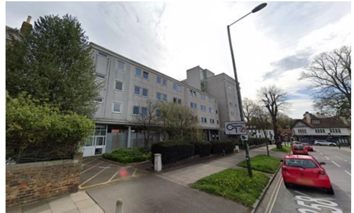
Elevation onto Grove Avenue
