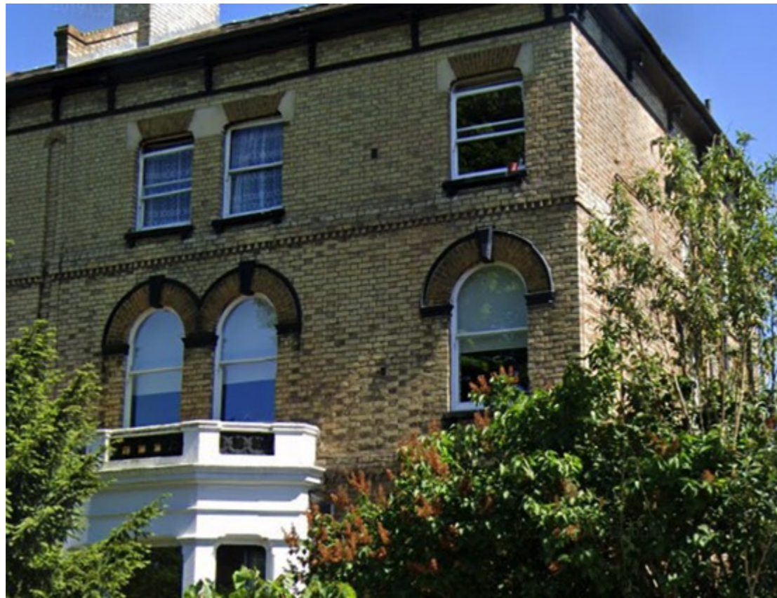
Yellow brick window surrounds and details.
