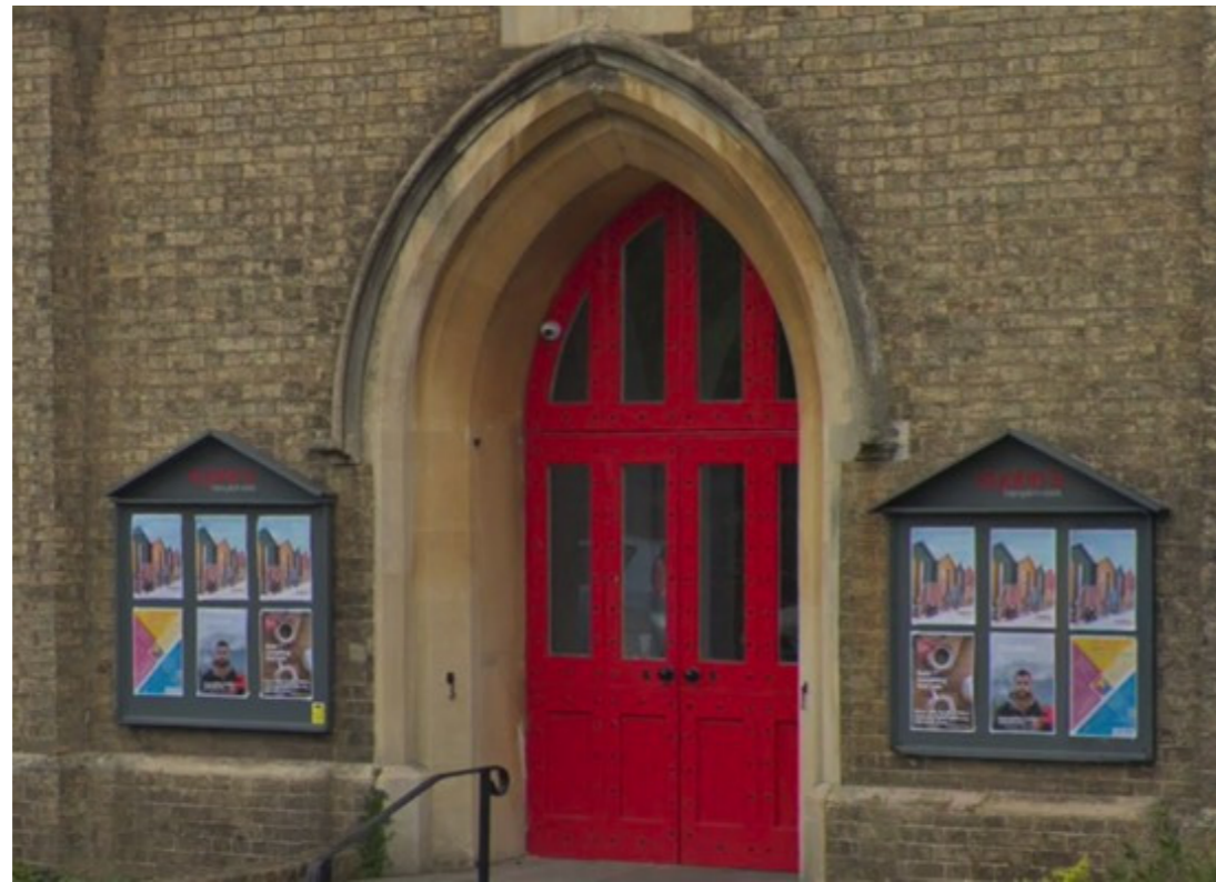
Stone arch and yellow stock brick church
