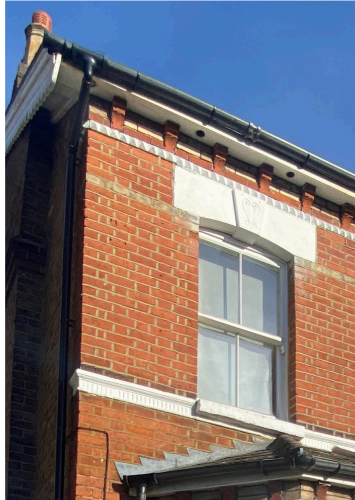
Brick detailing to front elevation
