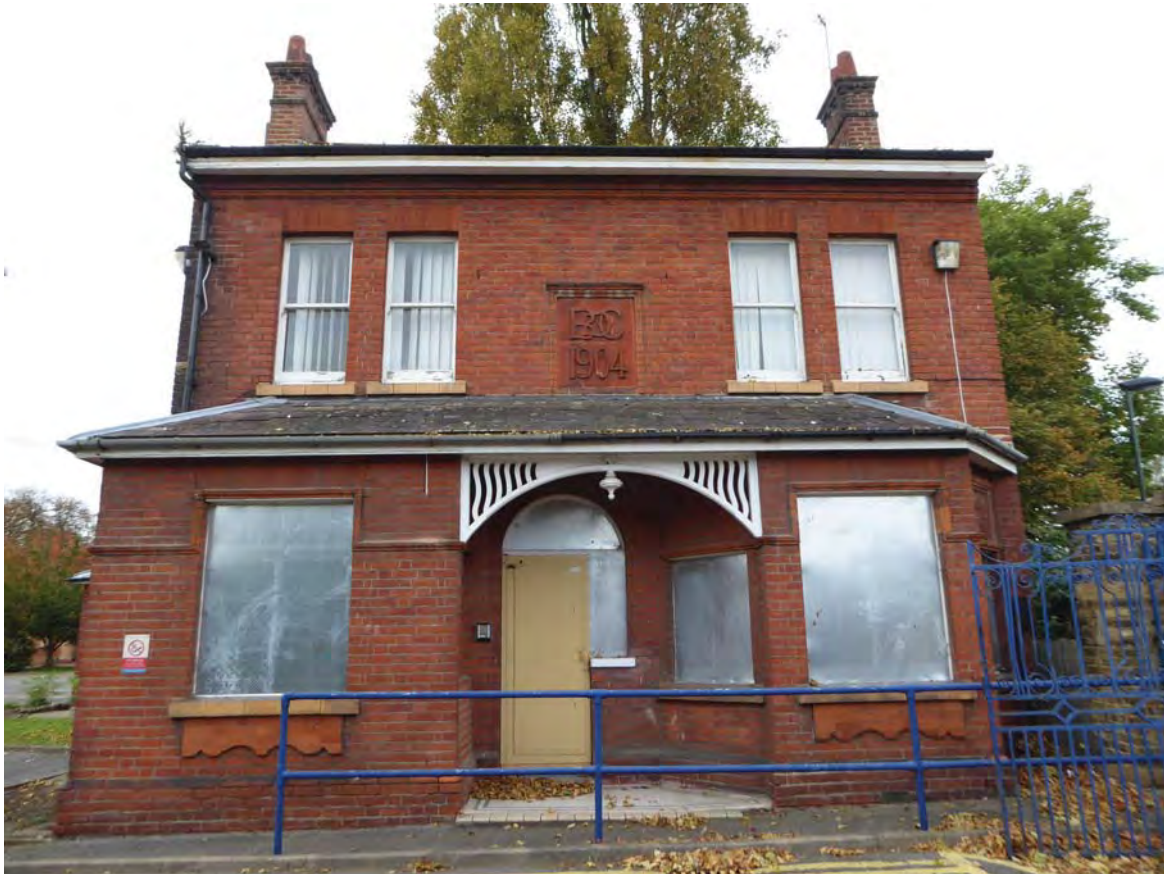
Plate 5: View east of Enid Balint Centre - 1904 building, Barnes Hospital
