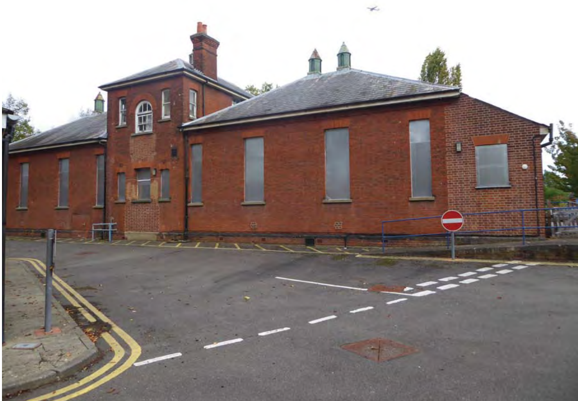
Plate 6: View south west of 1930s building, Barnes Hospital
