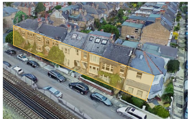
Figure 2: 1-15 North Worple Way windows
