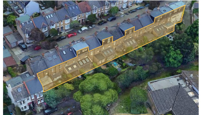
Figure 6: 2-26 Buxton Road windows
