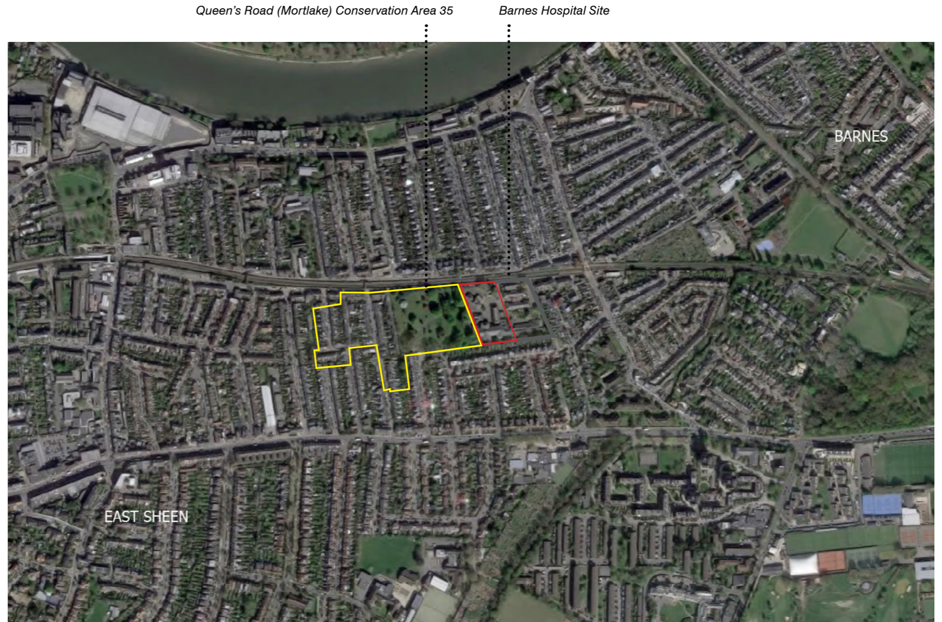
Barnes Hospital Site in Red, Queen's Road Mortlake Conservation Area in Yellow
