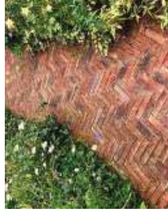
Reclaimed brick footpath
