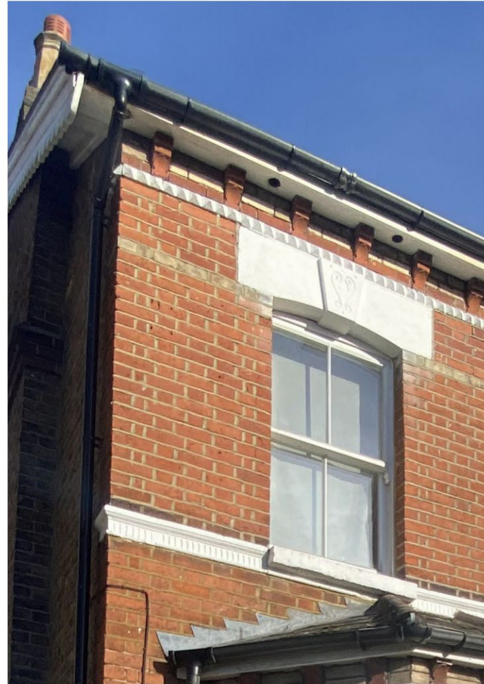
Brick detailing to front elevation
