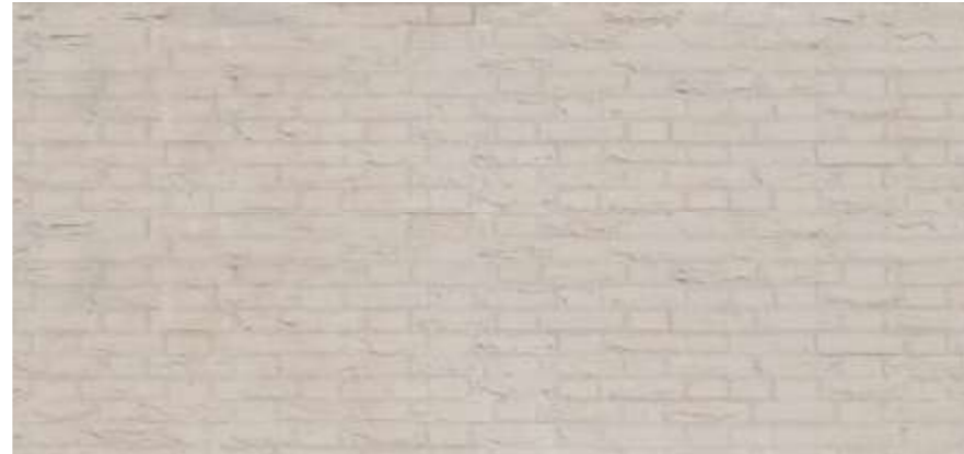
Pale Flemish bond brick walls
