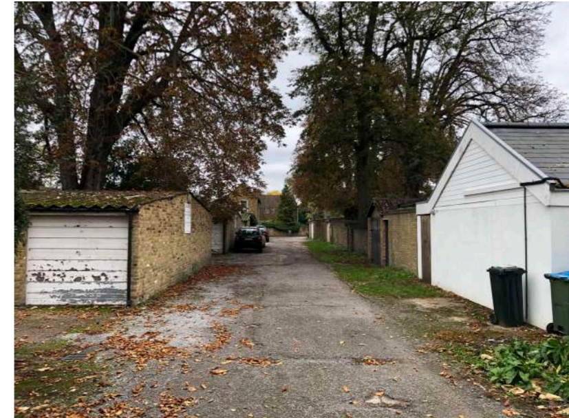
Fig.05 Driveway to rear of 37-49 Twickenham
