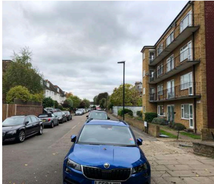
Fig.03 Manor Road, 35 Twickenham (flats)
