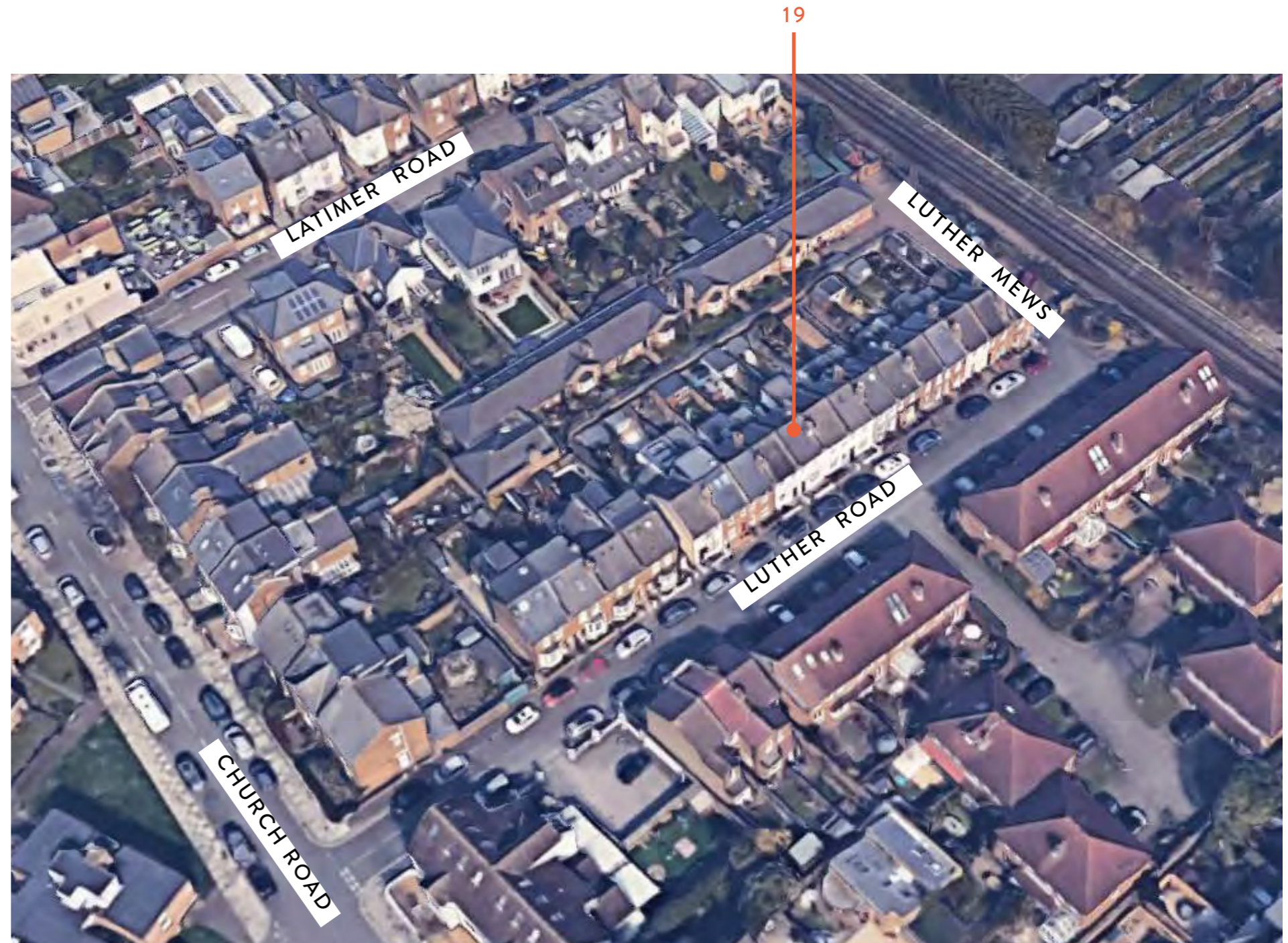
FRONT VIEW SOURCE: GOOGLE EARTH MAPS
