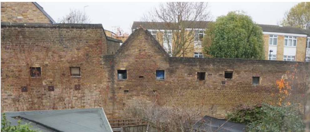
19 th century rear walling
