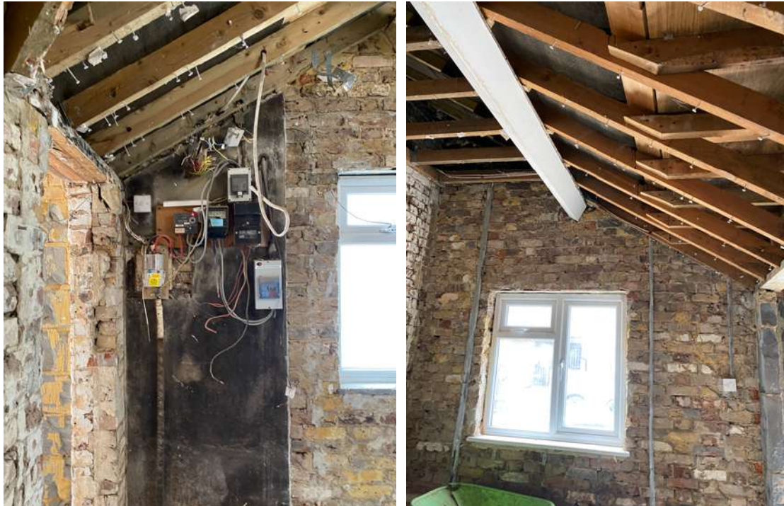
The internal faces of the front gable wall, with modern eaves rafters.
