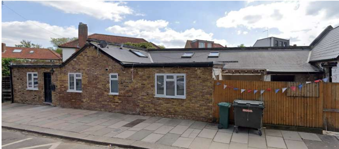
Residential building (left) with L shaped roof (centre) leaning on the top of the rear wall of the site.
