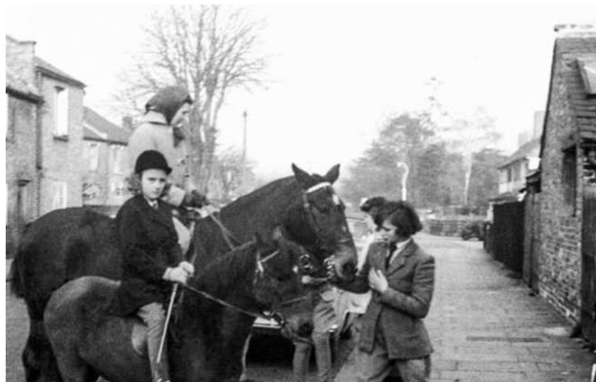
A 1960s photograph showing to RHS the above gable at that time, with side window and without flat-roof elements
