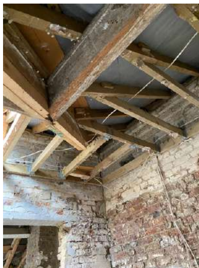
Old purlins supporting the pitched roof.
