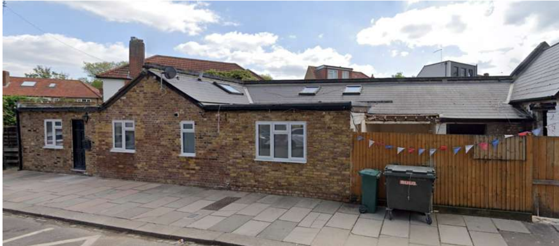
Residential building (left) with L shaped roof (centre) leaning on the top of the rear wall of the site.
