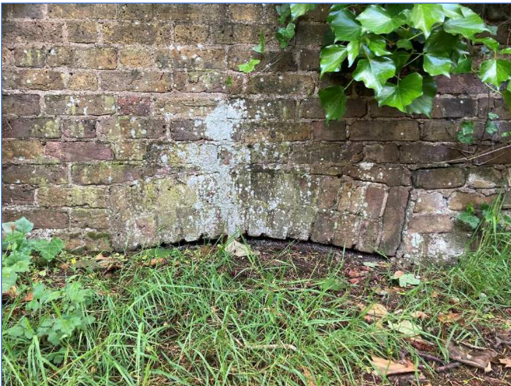
Plate 16: Southeast-facing detail of segmental arch at base of boundary wall / remains of structure near the south end of the eastern boundary of the Site
