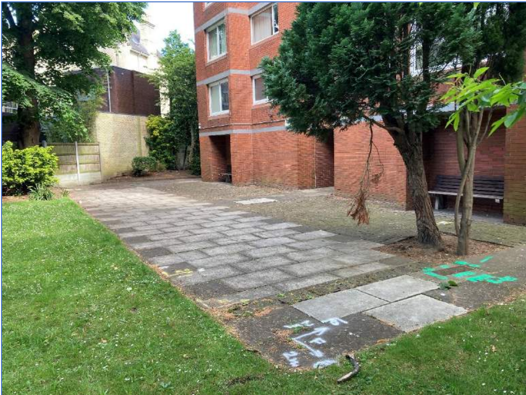
Plate 4: North-facing view of paving at the rear of Sheldon House
