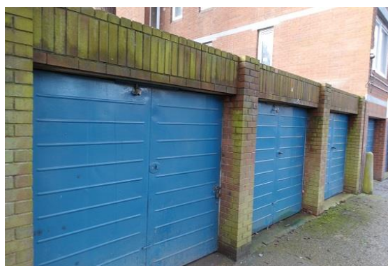
Plate 4.2: Garages on the Eastern Elevation
