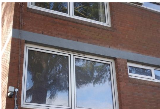
Plate 4.5: Weep Holes Above Window Lintels
