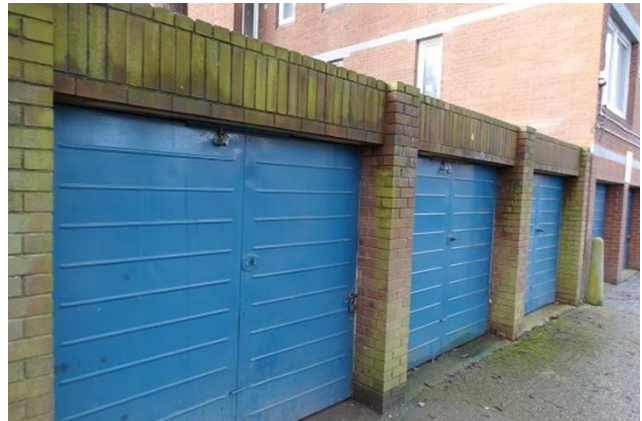
Plate 9.4: Garage terrace adjacent to the flat block
