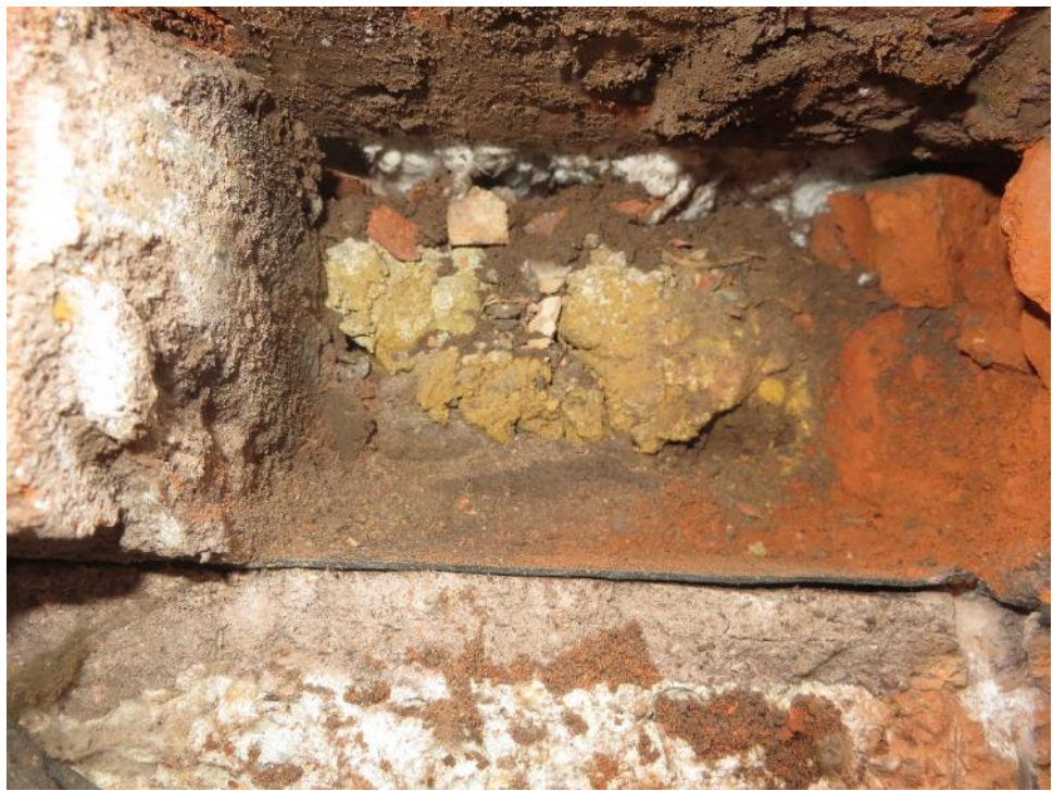
Debris and mortar above the cavity tray
