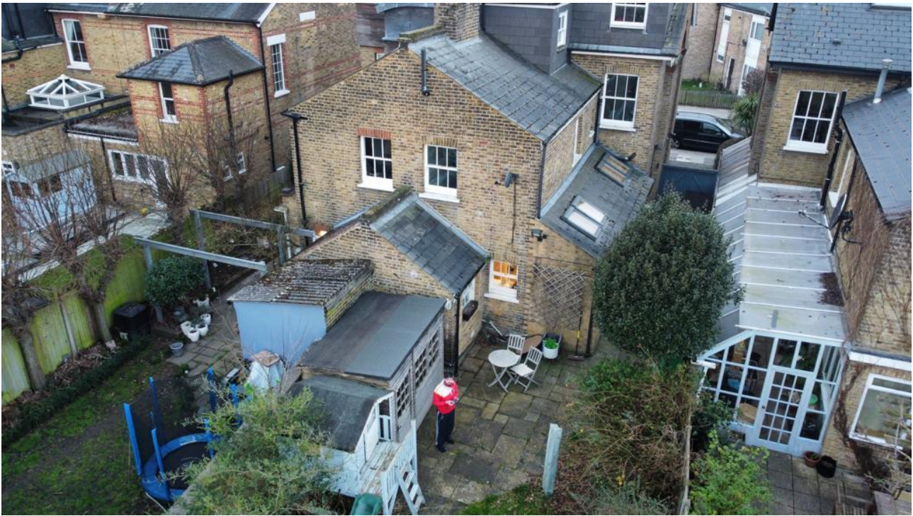
Fig 2. As existing aerial view of rear of No.62 (centre) and No.64 (right).
