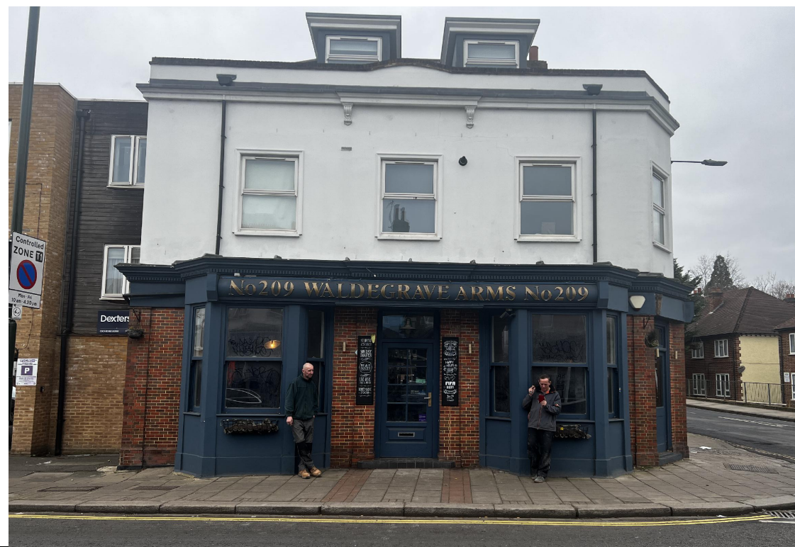
EXISTING SHOPFRONT - FRONT
