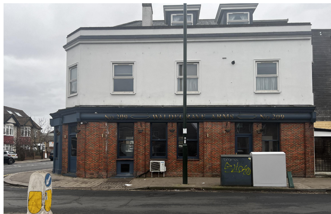
EXISTING SHOPFRONT - SIDE
