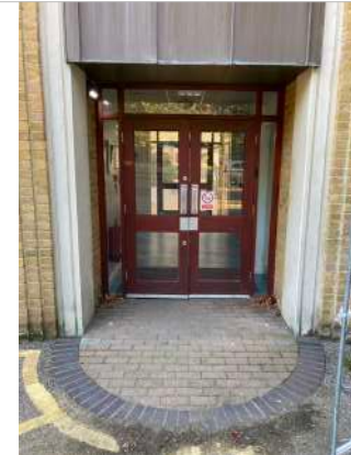
West Elevation entrance to Blocks M & L
