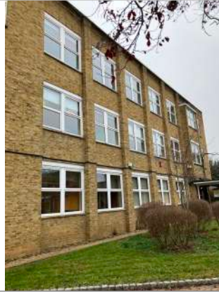
View of East Elevation
