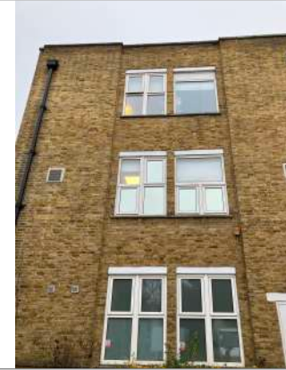
View of North Elevation
