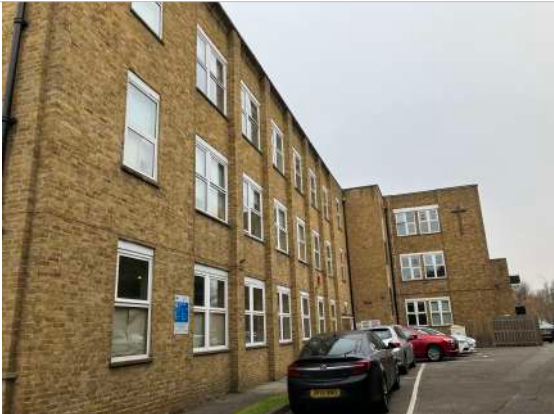
View of West Elevation
