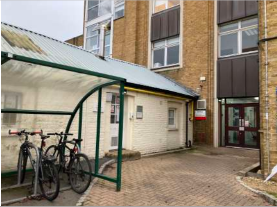
East Elevation entrance to Blocks M and L
