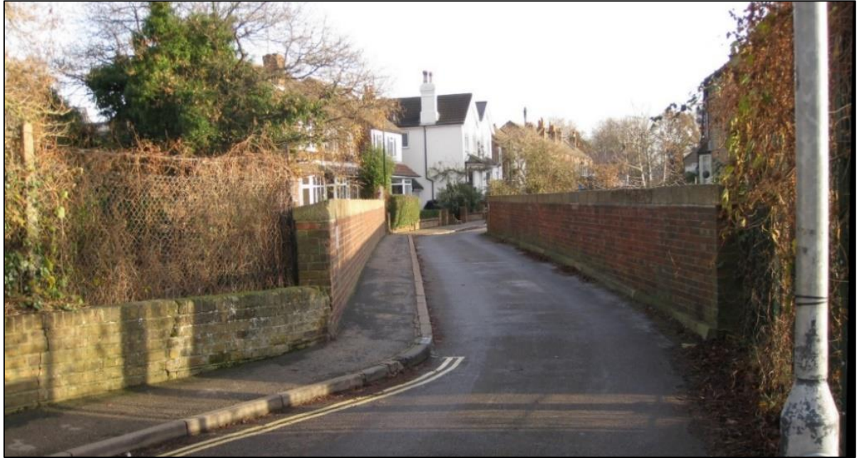
Figure 2.4 - Railway bridge between Holly Road and School Avenue
